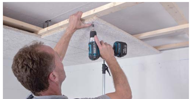
Install the acoustic tiles with the aid of a support. When fixing, press the tile onto the batten using the heel of your hand. There must be no gap between the tile and the wooden batten. For large ceiling areas, begin tile installation from the centre of the room. Observe the installation direction of square tiles!
