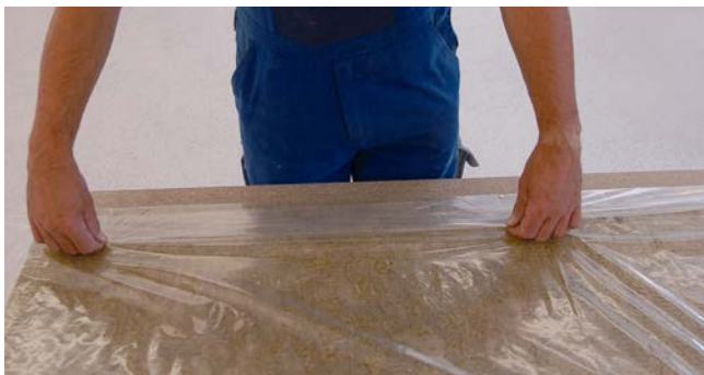
Fold over the film edges.
