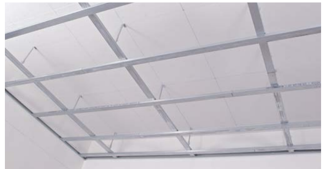
Finished ceiling grid.
