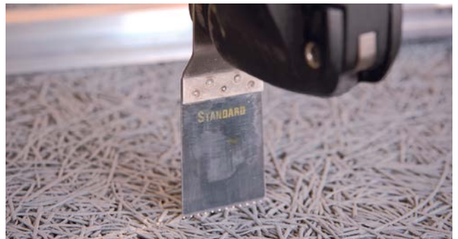
Cutting openings with a "supercutter" Only cut at a right angle to the tile surface.
