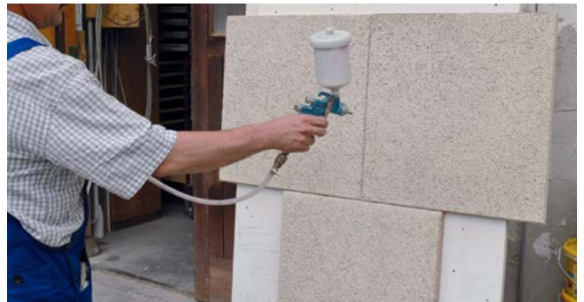
Painting or re-painting: The paint is sprayed on carefully with a spray gun using various spraying angles.
