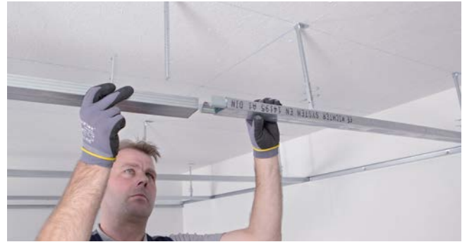
The CD-profile joints should be staggered. An additional hanger at every profile joint.
