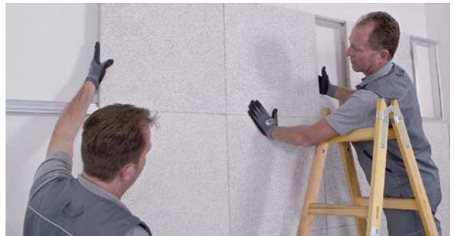
Slide in the tiles from the side. The edge profile of the last field is installed after tile installation.
