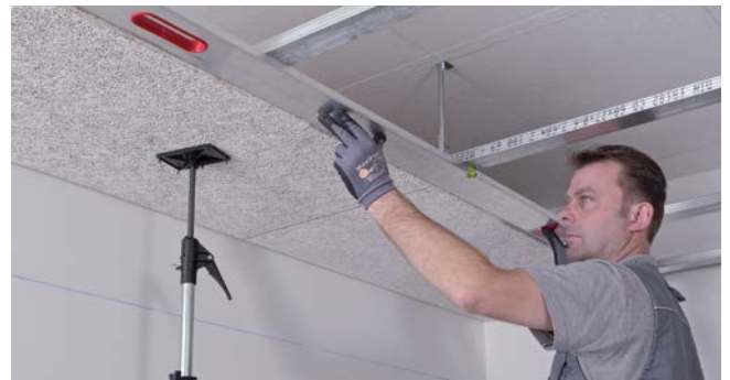
Align the rows of tiles with an installation batten. Tile joints must be positioned centrally under the profiles. No free tile joints are allowed! When installing square tiles, observe the installation direction marked on the back of the tiles.
