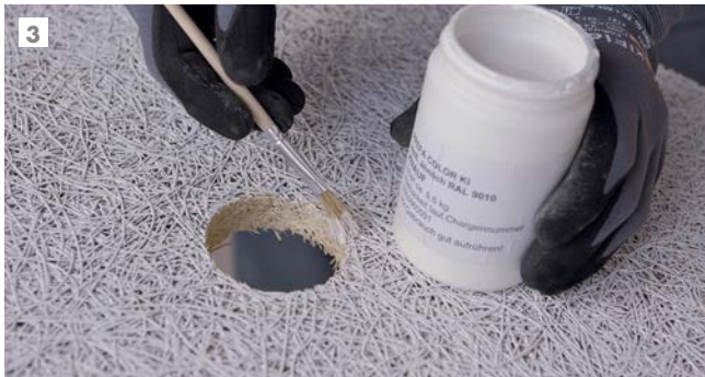
Cover cut edges with paint if these are not concealed by a cover.
