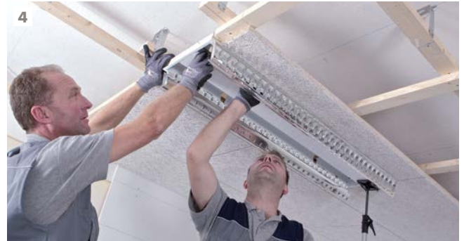
4 Alternative: Fix the ceiling light using screws into the wood battens or SD profiles at the sides or direct attachment into the ceiling.
