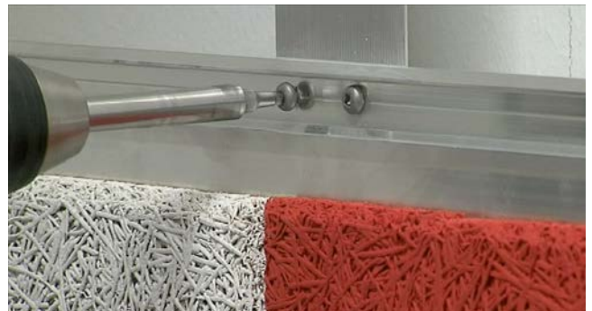
Fix the main profile with two self-drilling screws, 4.8 x 20 mm, per primary profile. Set the first self-drilling screw near the corner of the primary profile.
