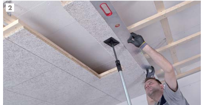
2 Installation of edge strip
