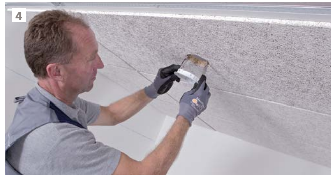
Insertion of the spotlight housing.
