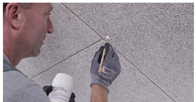
If coloured screws are not used, paint over the screw heads with the paint supplied or a suitable equivalent using a fine brush and suitable amount of paint. Screw heads must be flush with the tile surface.
