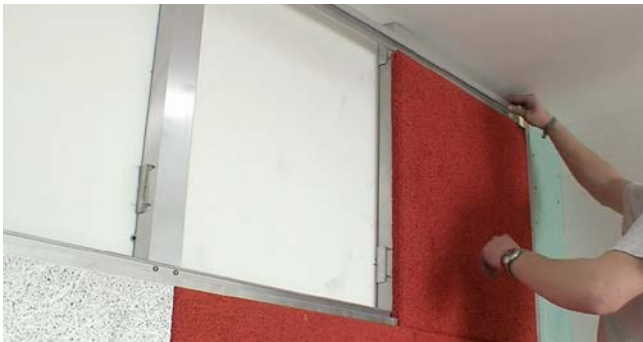
Installation of the upper edge profile. Space required from the ceiling approx. 40 mm. The first tile is moved approx. 10 cm towards the middle, the screws are fixed and then the tile is finally aligned in the grid.
