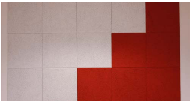
Lay out the profile centres from the middle of the room taking into account equally sized perimeter margins and the maximum permissible centres.
