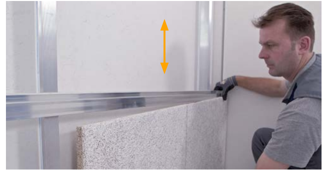
Fix the main profile at the end with only one screw so that the other end remains adjustable. This makes inserting further tiles easier.
