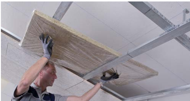
Insert HERADESIGN® acoustic overlays or other acoustic overlays, step-by-step when installing the HERADESIGN® acoustic tiles. Absorber tiles that are pushed between the CD-profiles are cut to size.
