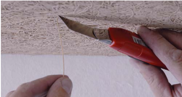
Dangling fibres: Carefully remove individual loose fibres with a knife.
