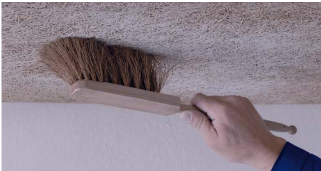
Brushing: Efflorescence, dust, etc. can be removed with a soft brush. Set loose fibres with StoPrim Plex primer.
