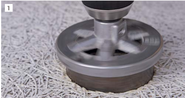
Drilling of a round aperture for a spotlight, with tile face side up.
