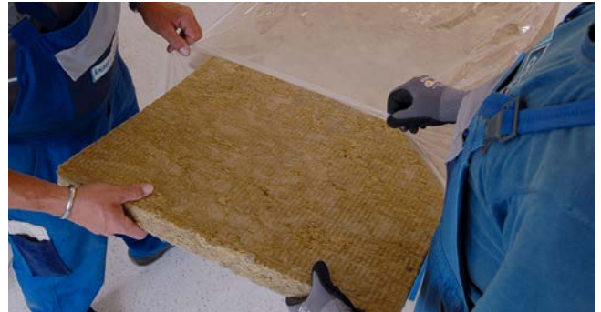
Slide in the acoustic overlay.
