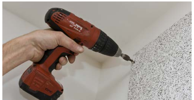
If there is no space to move the tile across, fix the last tile by means of a screw. Cover unpainted screw heads with paint in the colour of the tile using a fine brush.
